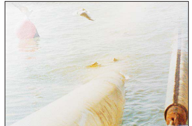
Lowering one end of the pipestring by means of a stringer.
