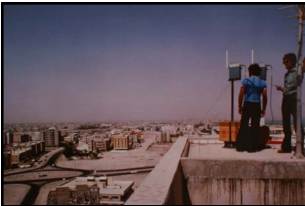
Installation Decca Trisponder in Salmiyah und Calibration Check Landing Point Failaka
